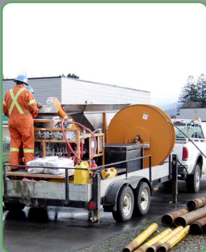
■ Grouting of geo loop.
