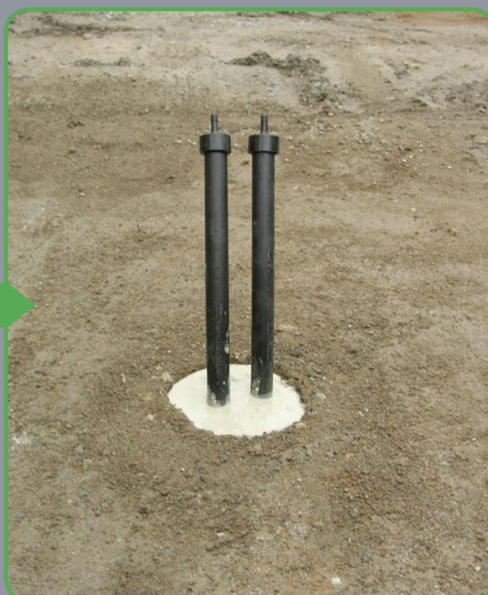
■ Completed geo loop installation.
